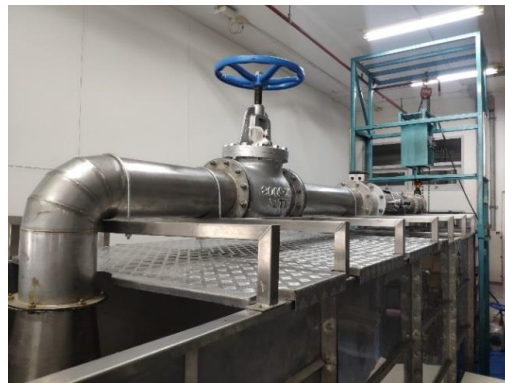
Figure 5. Photograph of pump performance test rig
