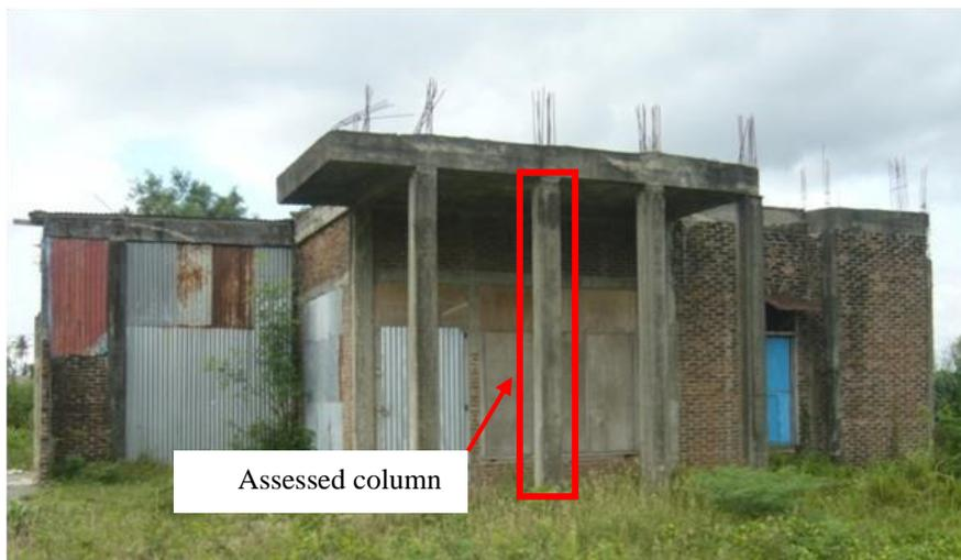
**Figure 3.** Residential reinforced concrete building which was affected by 2004 tsunami Sumatra
