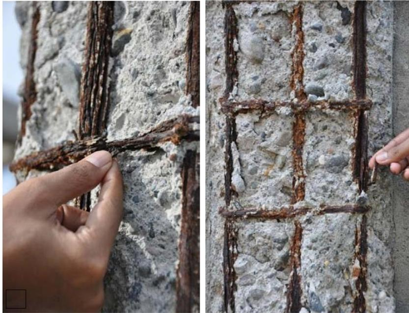
**Figure. 12.** The worst actual corrosion of rebar after reconstructed for actual condition prediction
