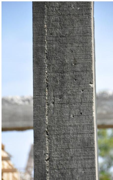
**Figure. 9.** The current assessed concrete cover condition during field assessment
