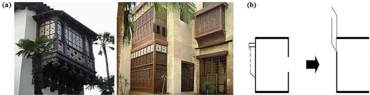
Figure 7. (a) Takhtabush in an old Egyptian house and (b) New model is based on the geometry and position of Takhtabush
