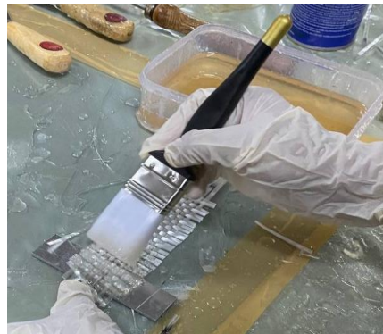
Figure 3. Layering process of composite material on a cracked plate
