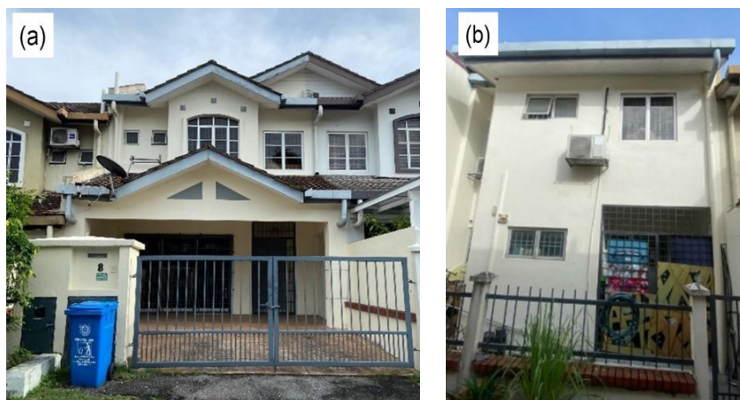
Figure 2. Pictures of a single unit terrace house in (a) front view and (b) rear view
