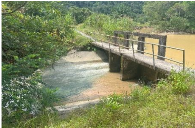
Figure 2. Irrigation pond and dam
