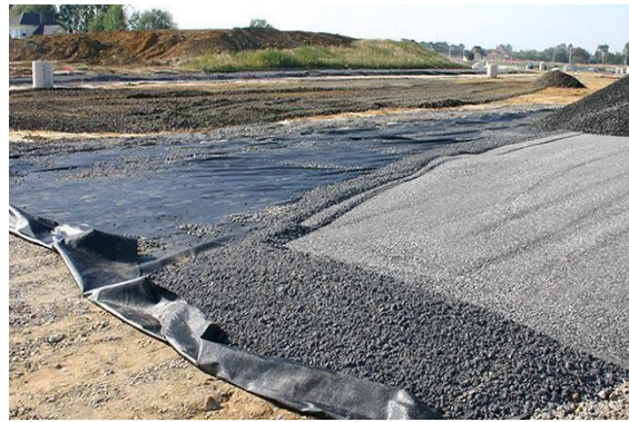
Figure 3. Geotextile material at site
