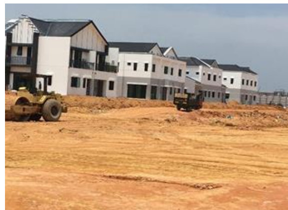
(b) Show houses nearing completion
