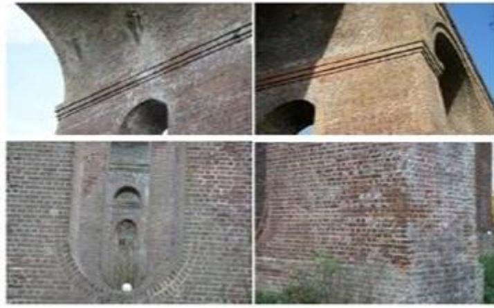
Figure 8. Samples of images of the Chapel viaduct.
