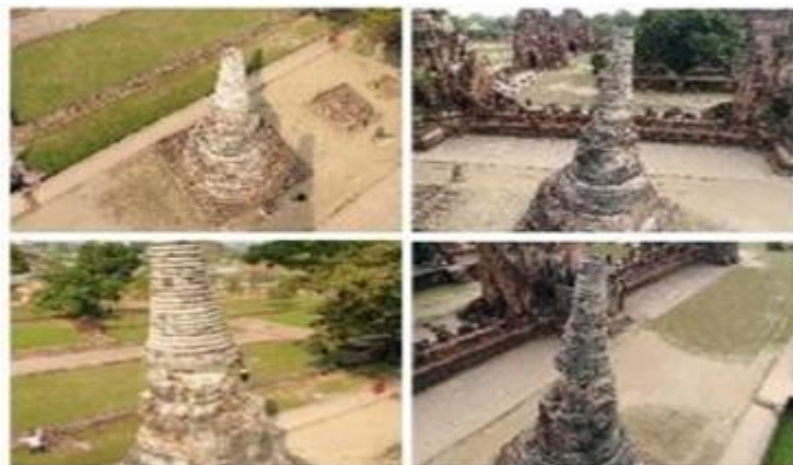
Figure 7. Sample images acquired using a UAV.
