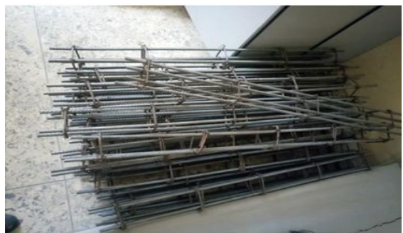
Figure 4. Reinforcement bars with shear links
