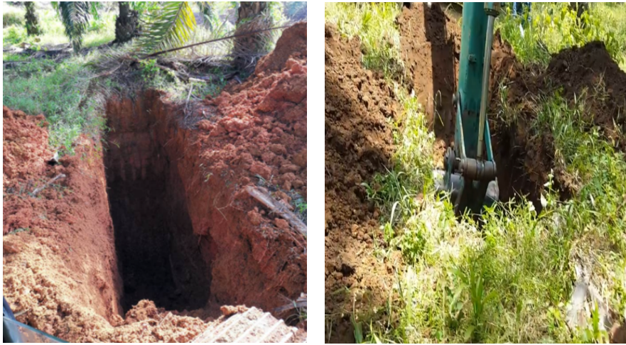
Figure 6: Site Photography showing trial pit at site
