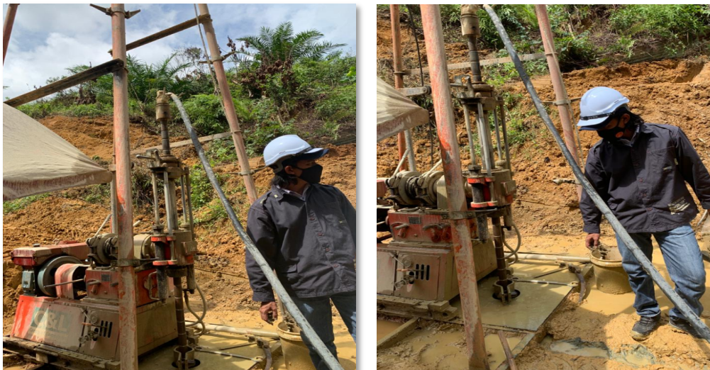
Figure 7: Site Photography showing Bore Holes Diamond Driller
