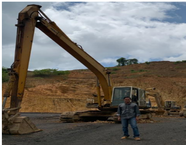
Figure 5: Site Photography showing Hydraulic Excavator 350 Komatsu
