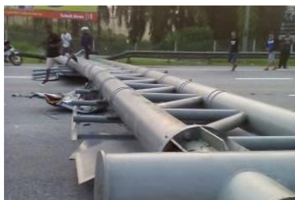
Figure 3: A signboard girder collapsed onto a passing car
