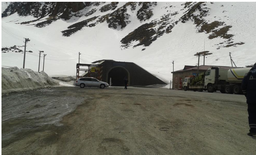
Figure 1. Too-Ashuu Pass (Northern side of the K. Kolbaev tunnel, altitude 3120 m above sea level)
