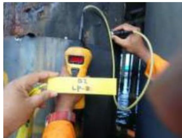
Figure 1. Ultrasonic wall thickness testing for above water pile
