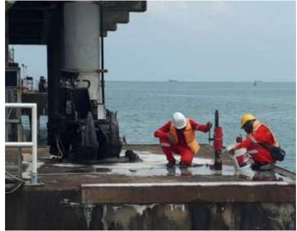
Figure 5. Concrete coring (100 mm \phi x 150 mm length) for compressive strength test
