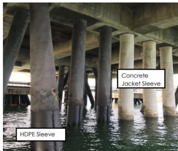
Figure 14. Concrete jacket sleeve and HDPE sleeve
