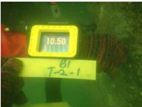
Figure 2. Ultrasonic wall thickness testing for underwater pile
