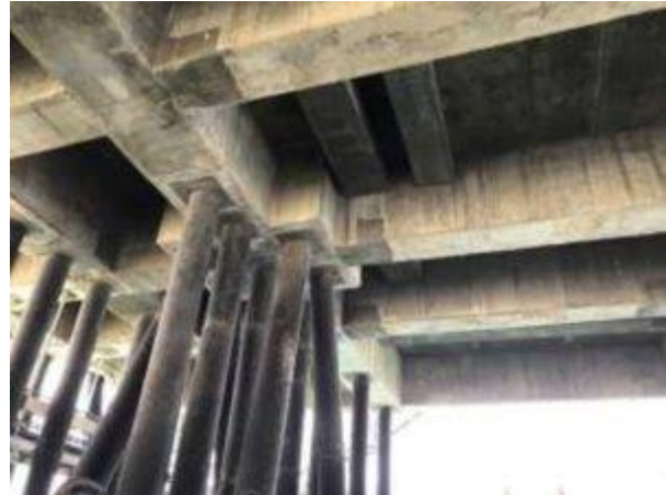
Figure 9. Under deck soffit (good condition)
