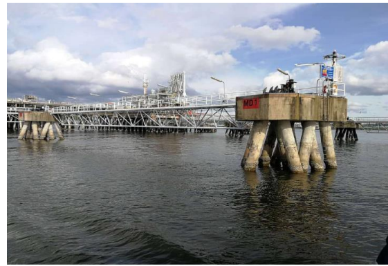
Figure 11. Catwalk between mooring dolphins is still in good condition
