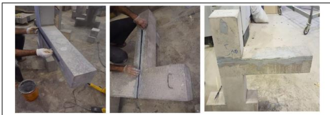
Figure 10. Creating grooves on the top of the beam and adding strips [1].
