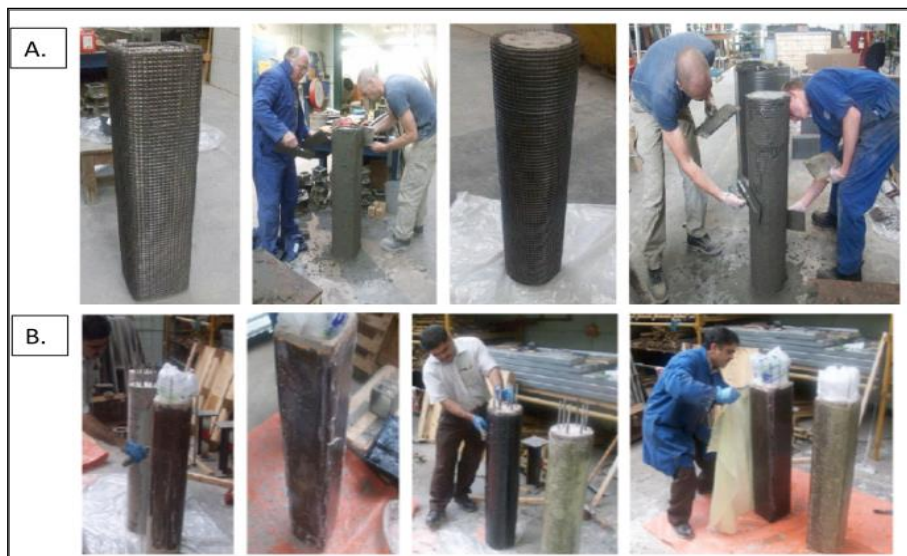
Figure 6. Repairing procedure application of (A) Ferro cement, (B) FRP jacketing [10].
