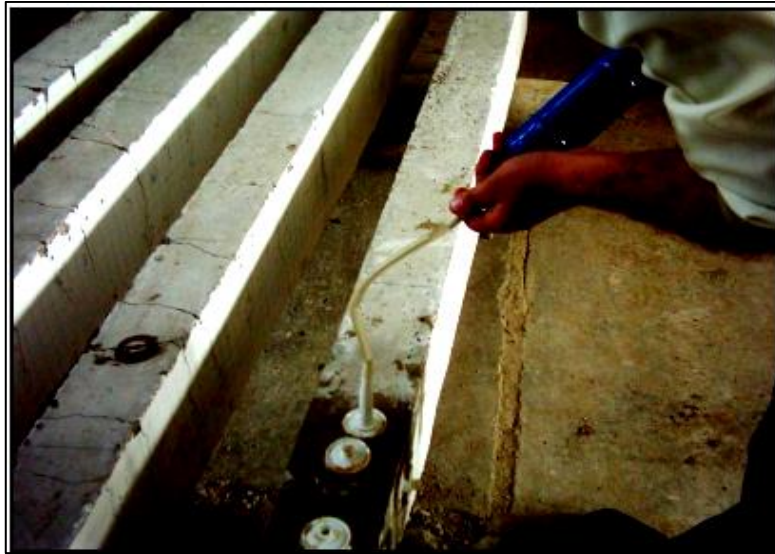
Figure 7. Epoxy injection for beams.
