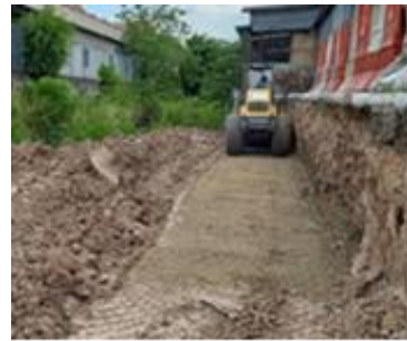
Figure 8. Compacting of granular fill
