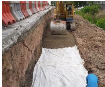
Figure 7. Filling of granular fill
