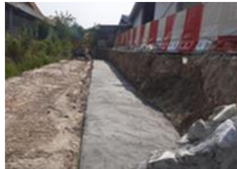
Figure 10. Casting of levelling pad
