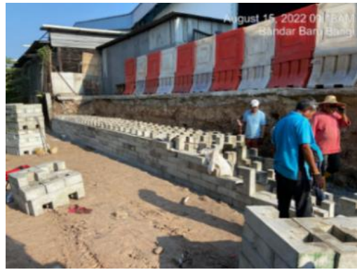
Figure 12. Laying of EC Geoblock
