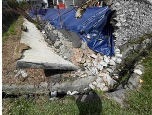
Figure 6. RC retaining wall failure
