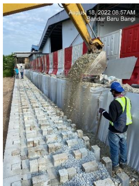
Figure 14. Backfill crusher run
