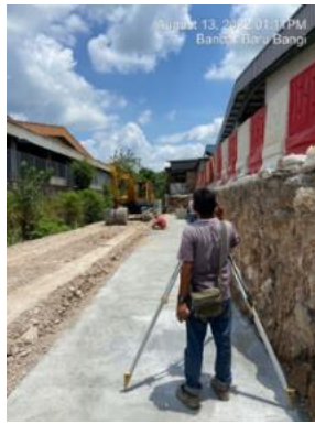
Figure 11. Alignment checking
