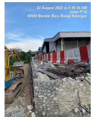
Figure 16. Construction of rubble wall
