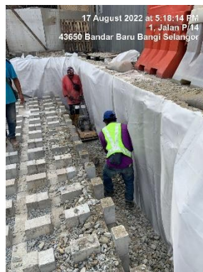
Figure 15. Compact crusher run
