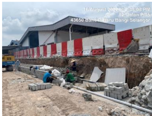
Figure 13. Subsoil pipe installation and laying of EC Geoblock
